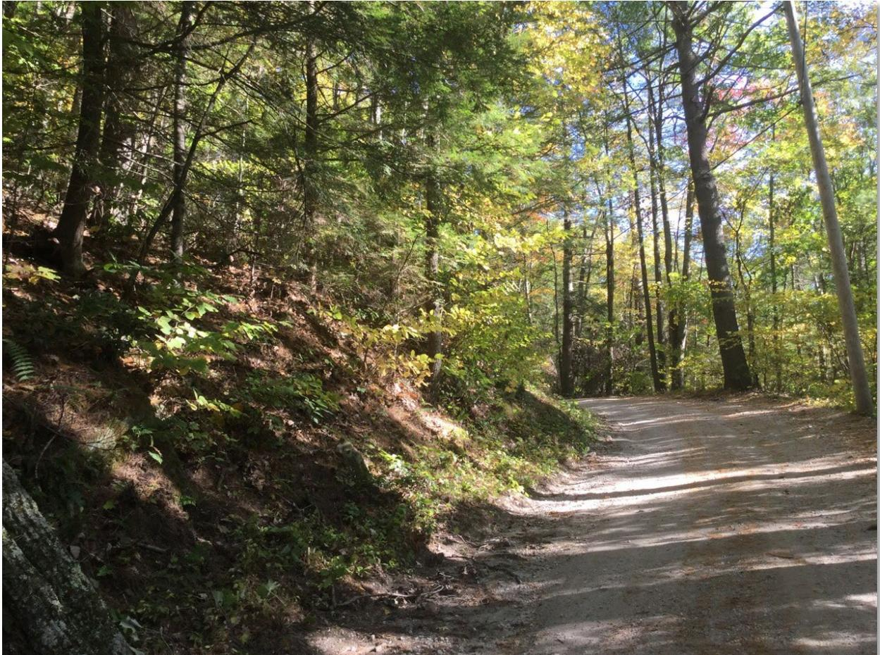
*Example of steep adjacent slopes and an in-sloping roadway crown on Campbell Falls Road, New Marlborough, MA*
